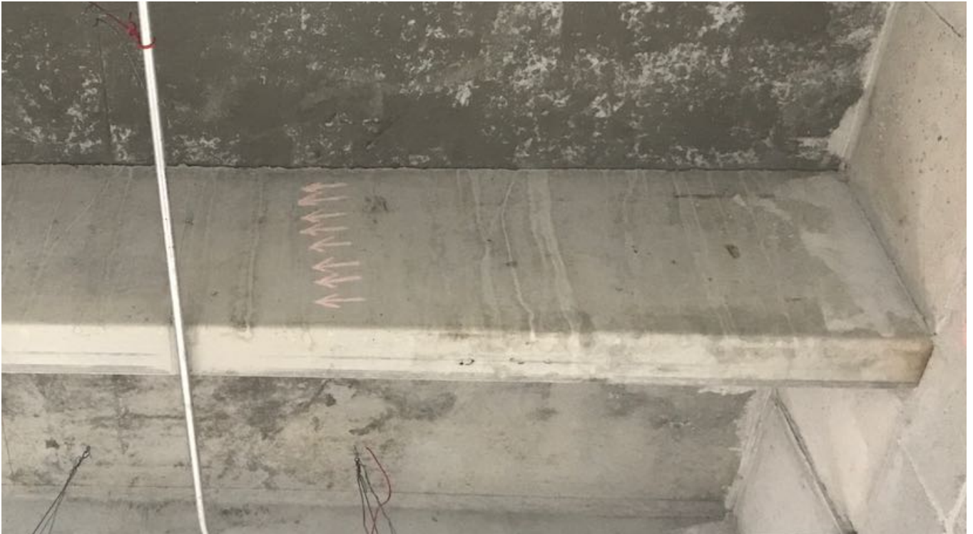
The mono wings have 8 cables that descend from the ends with profile to form a group at mid beam.
