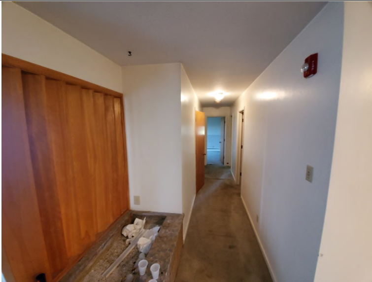
5) Hallway – Texture on walling material positive for asbestos.
