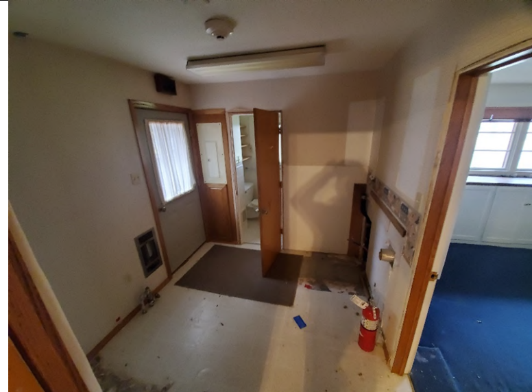
6) Utility Room – Texture on walling and ceiling material positive for asbestos.
