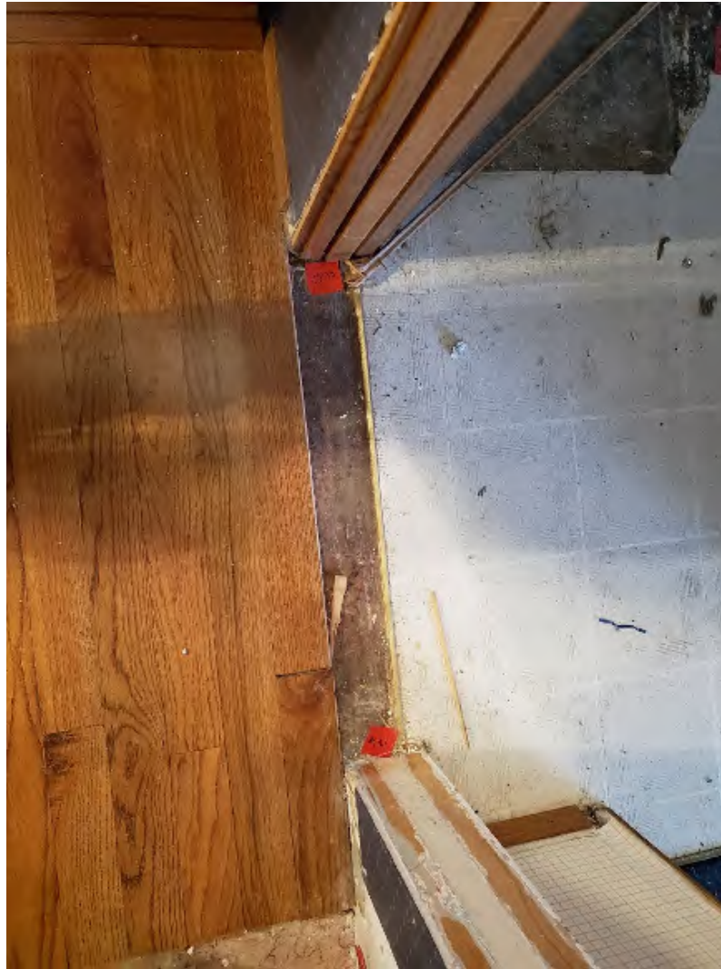
9) Kitchen – Paper backing under sheet flooring positive for asbestos (located under red floor tile).
