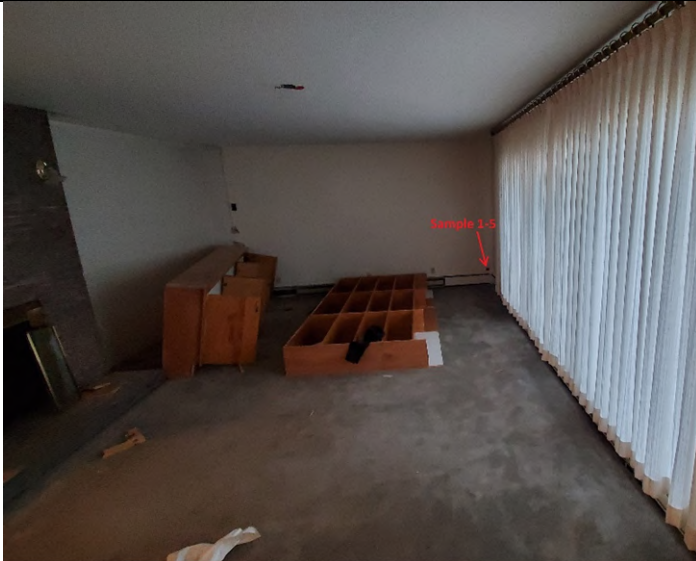
1) Living Room – Texture on walling material positive for asbestos.
