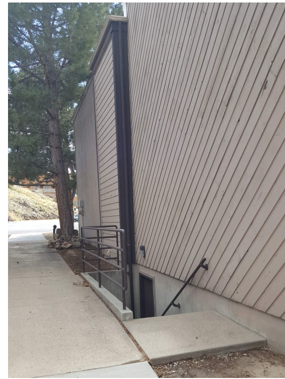
STAIRS AND RAILING AT BUILDING H
