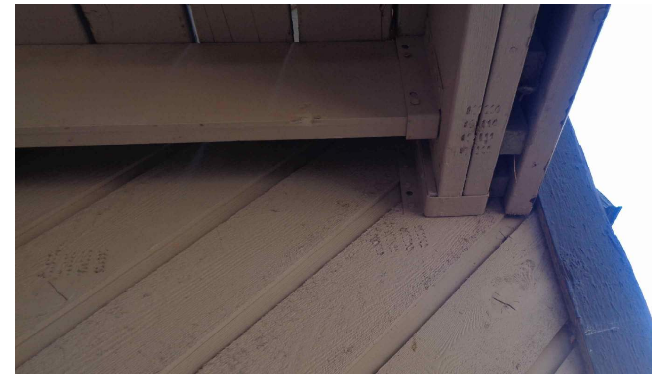
TYPICAL UNDER DECK/BOTTOM OF RAILING CONNECTION
