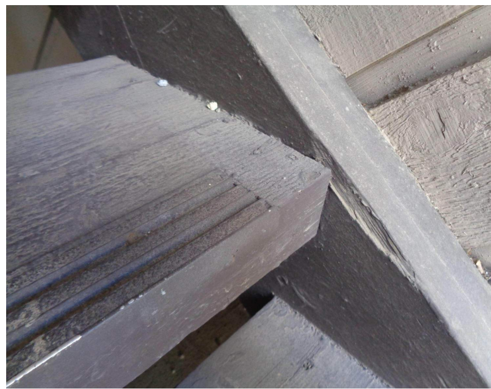
TYPICAL STAIR STRINGER TO WOOD SIDING CONNECTION
