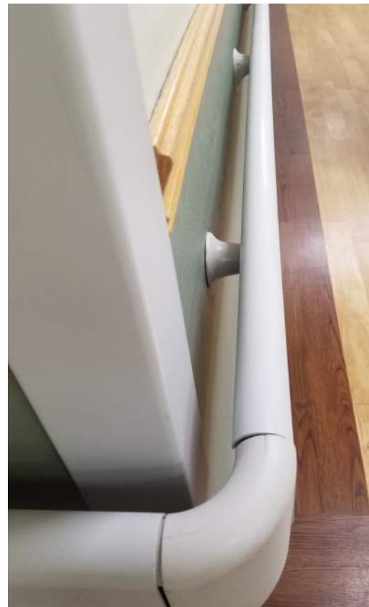
TYPICAL HANDRAIL ATTACHMENT
