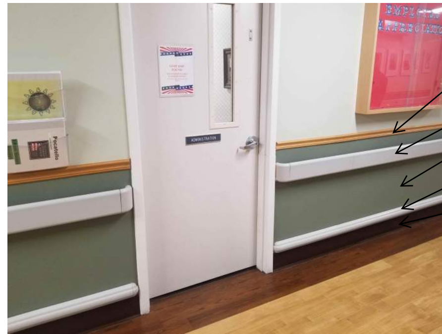
TYPICAL CORRIDOR CONDITION
