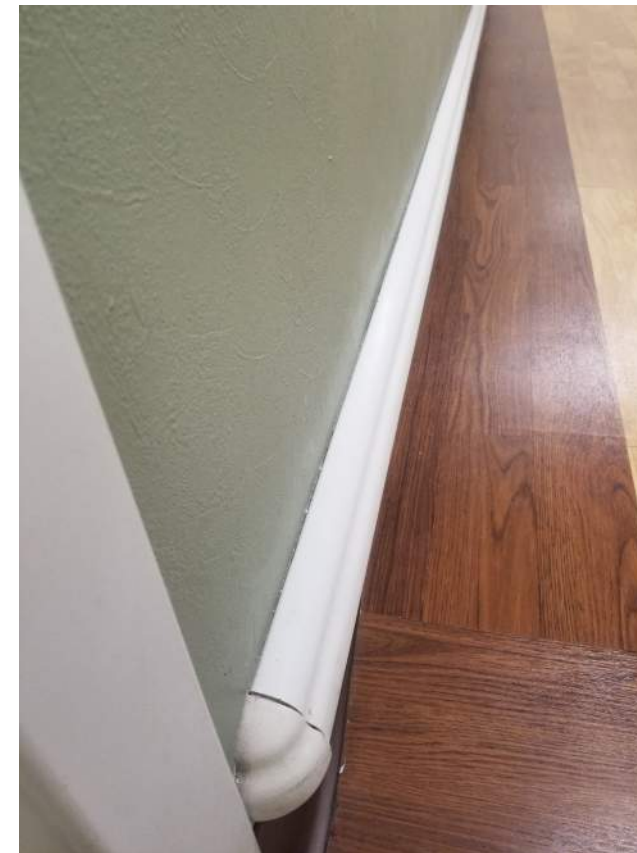
TYPICAL CRASH RAIL CONDITION
