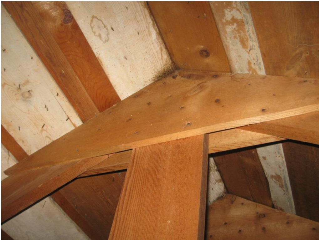
Photo 12 – Bearing site connection
