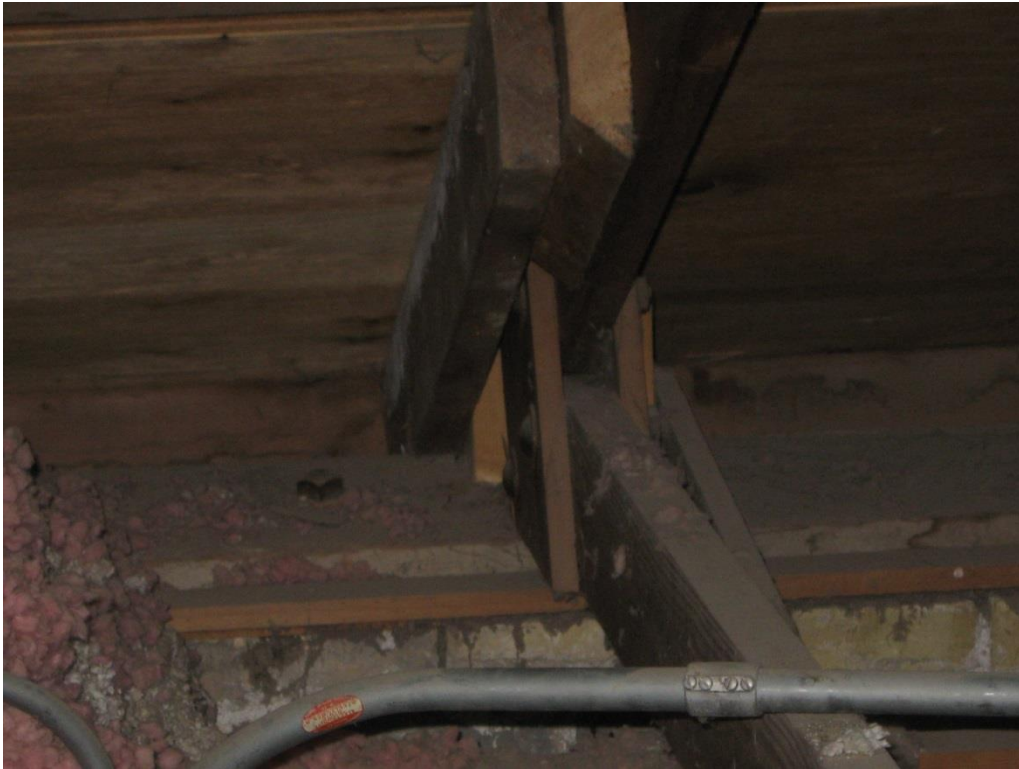
Photo 11 – Bearing site connection
