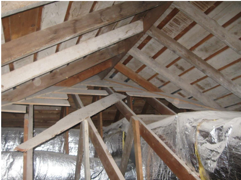
Photo 8 – Roof overbuild
