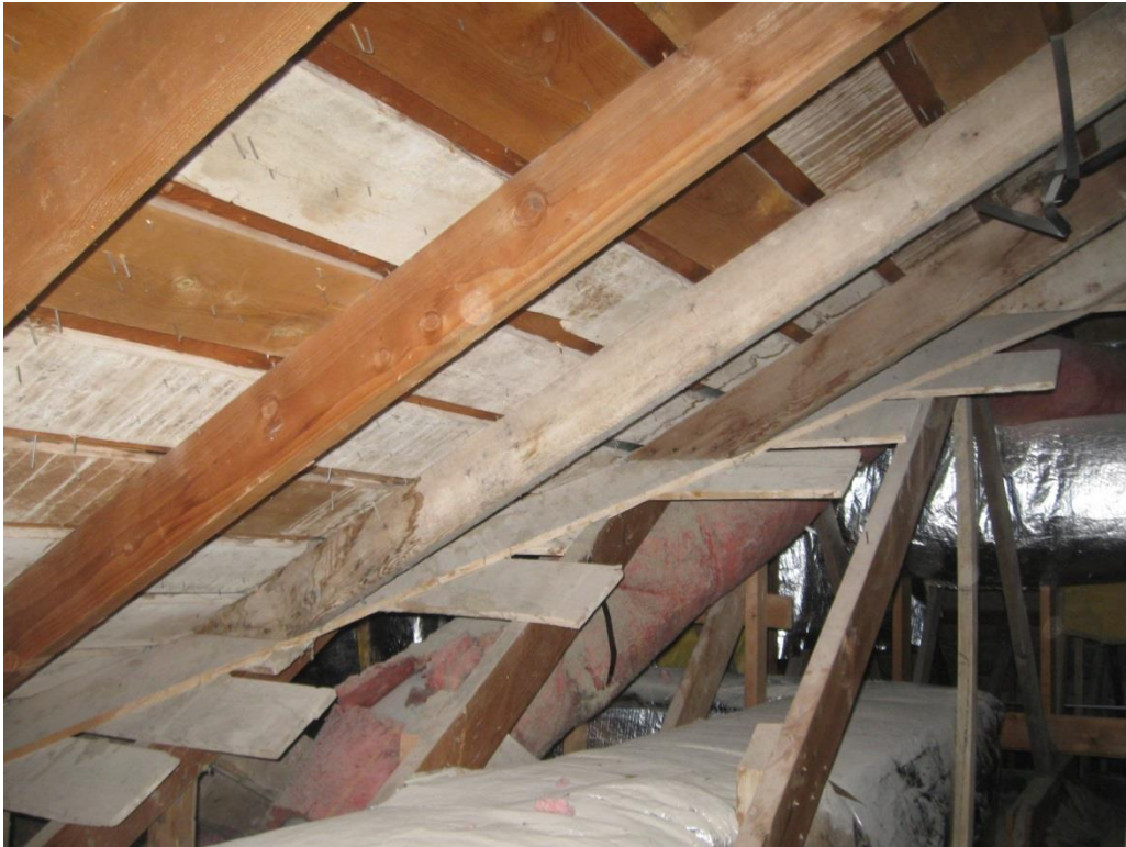
Photo 10 – Roof Overbuild
