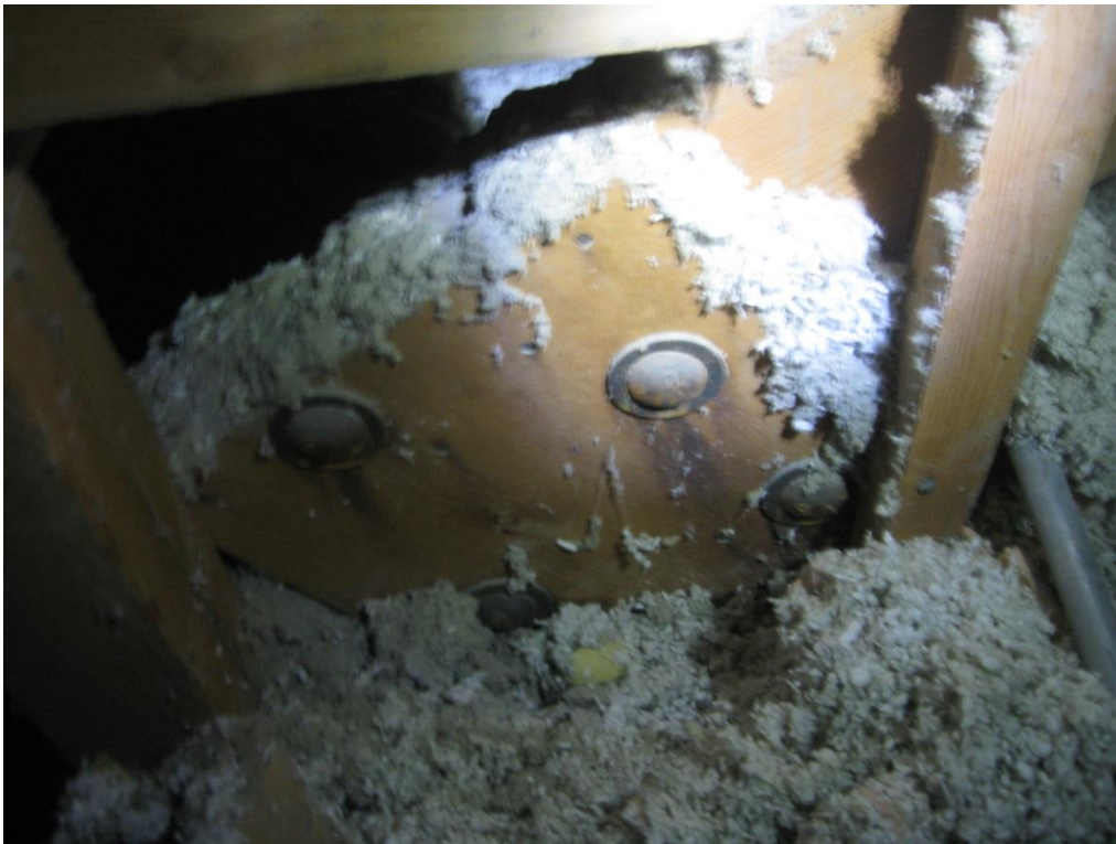
Photo 4 – Bearing site connection
