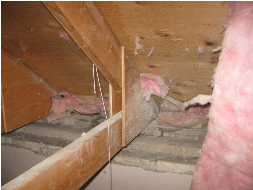
Photo 1 – Nailed bearing site connection
