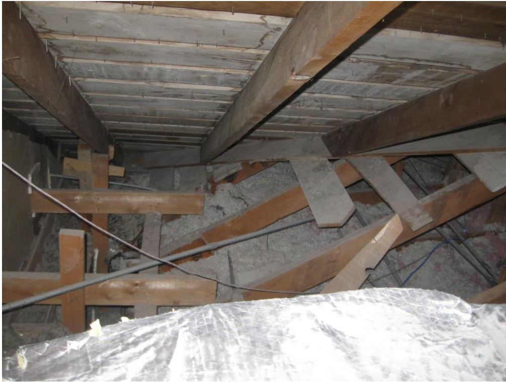
Photo 9 – Roof overbuild
