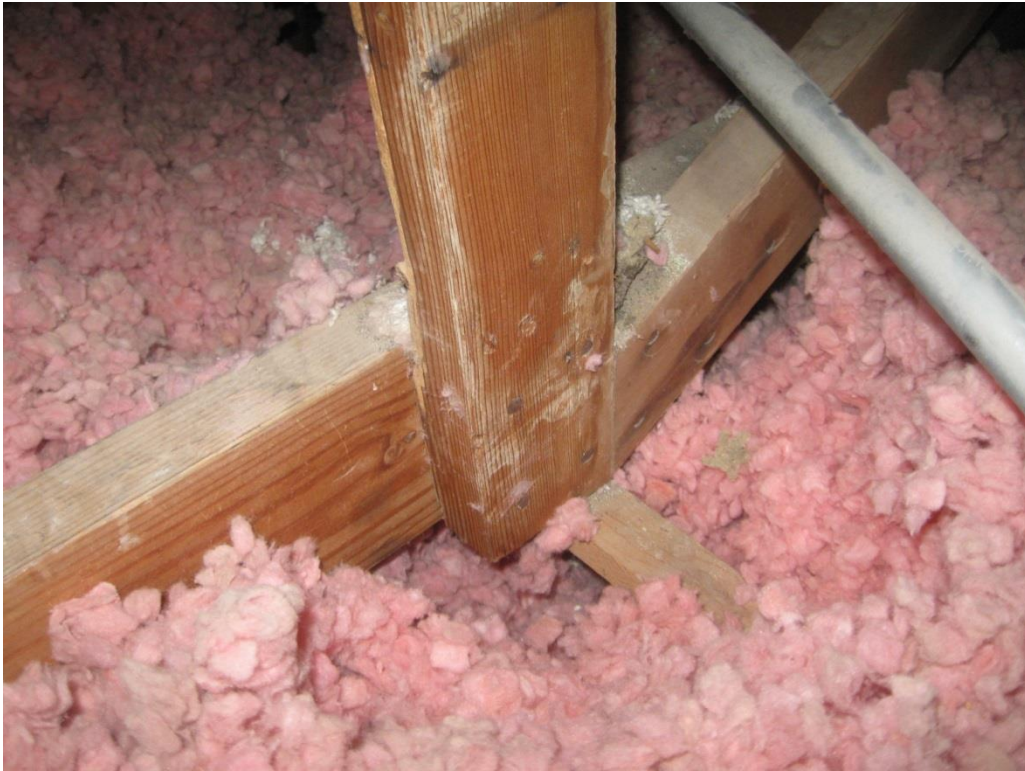
Photo 13 – BC to short compression web
