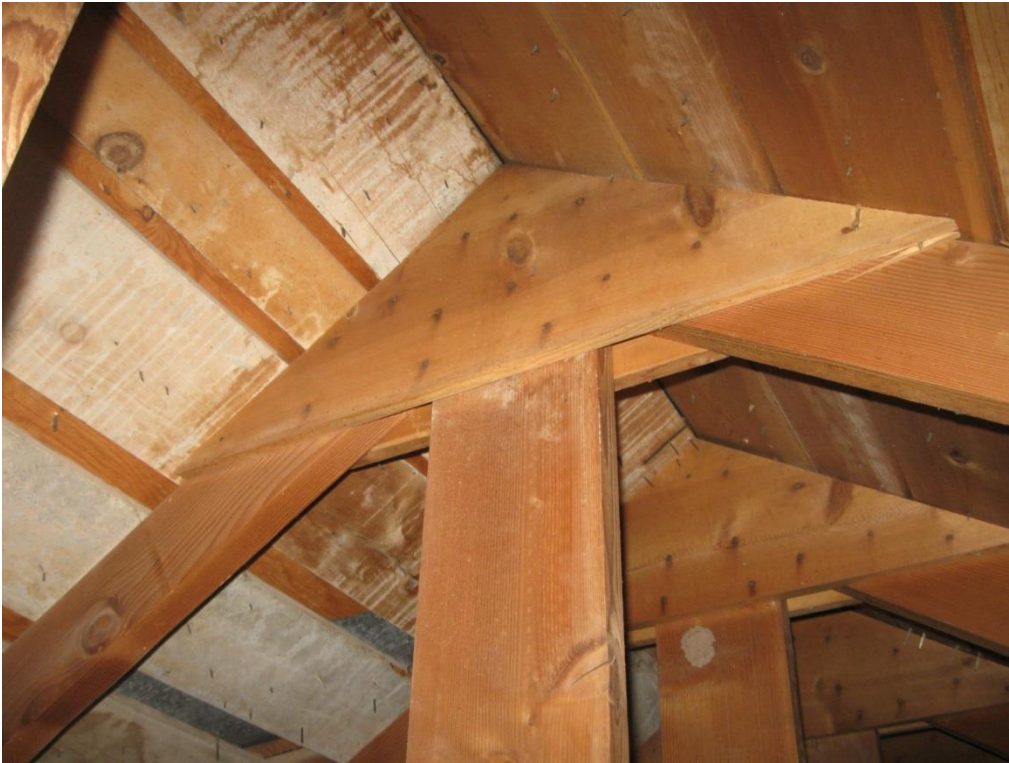
Photo 5 – TC and vertical web to gusset
